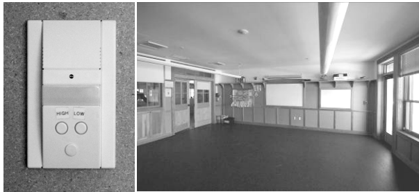
Figure 1: The triple level lighting control used in classrooms of Schlitz Audubon Nature Center.
